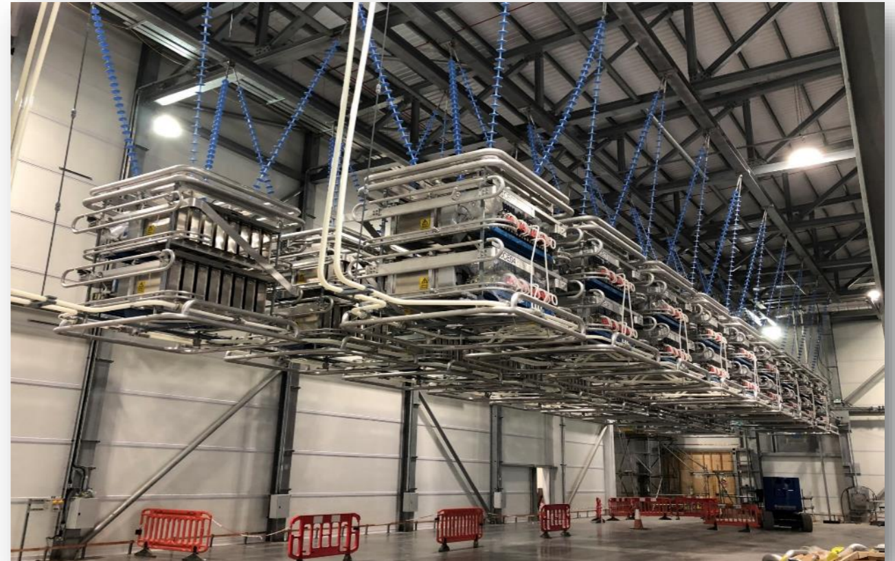
IGBT Valve installation at Spittal
